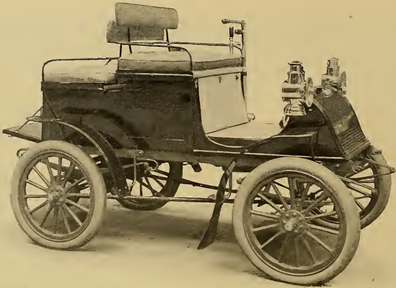
GASOLENE AUTO-CAR DOS-A-DOS OR GOLF TRAP, SPEED 8 TO 21 MILES—COST, $1,300.
